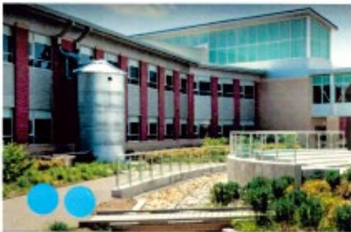
Energy and Water Efficient Architecture
