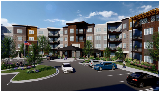
Class I materials: Multifamily Apartment
