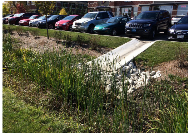
Parking Lot Stormwater
