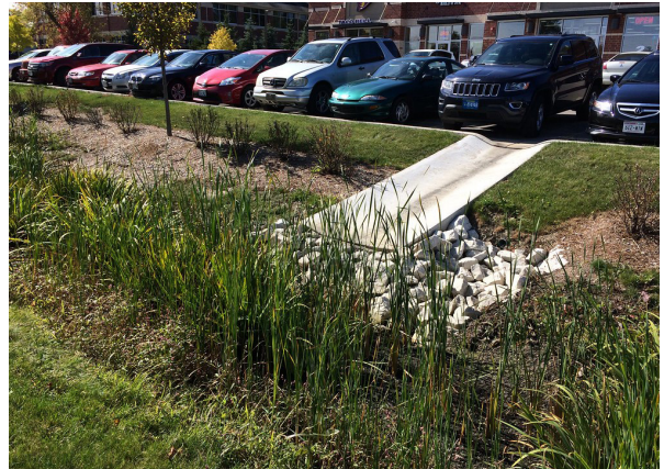
Parking Lot Stormwater
