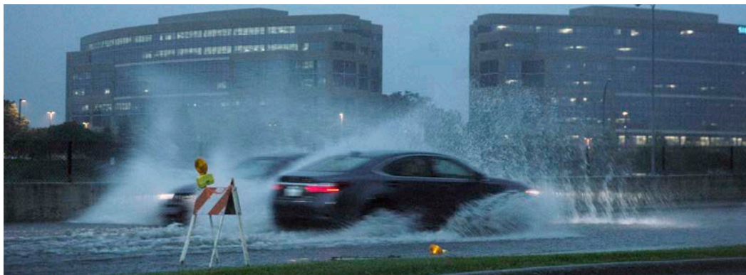
Localized urban street flooding, 2013
