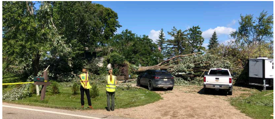
Surveying the damage from an EF-1 tornado in Minnetrista, 2019.
