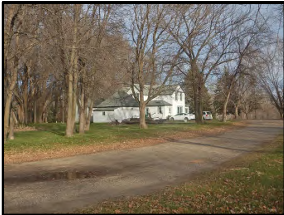
Figure 10. View of HE-COC-006 showing the rear of the building and remaining outbuildings.
