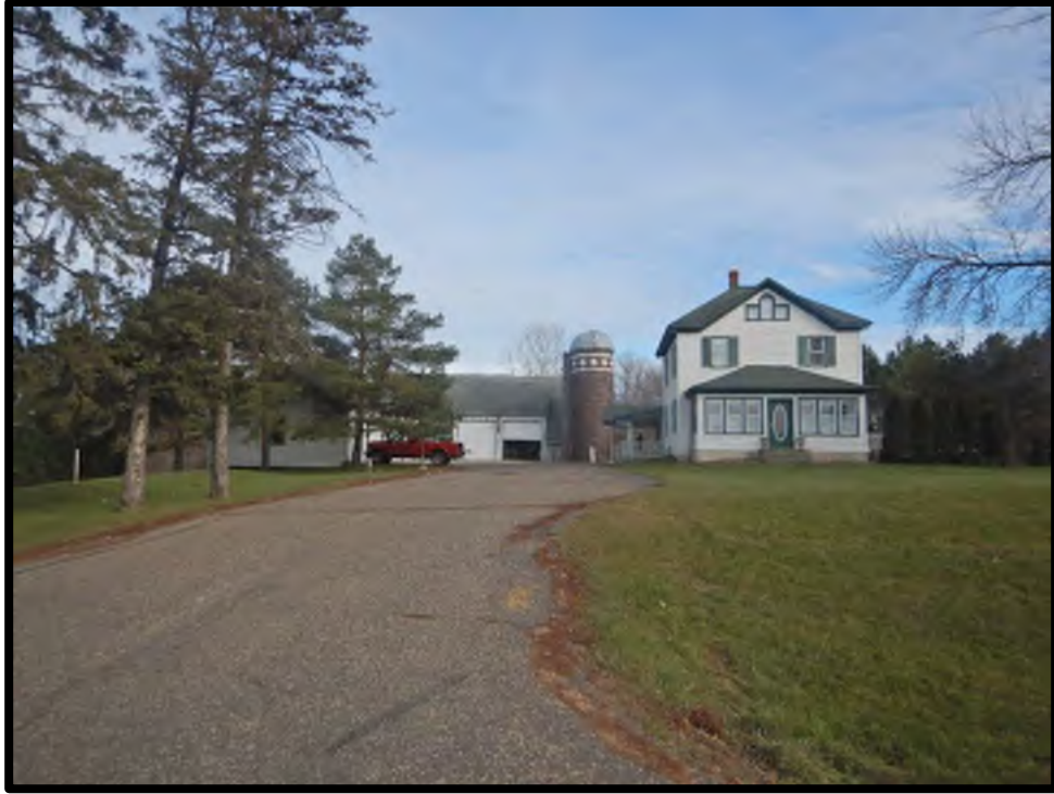
Figure 7. View of HE-COC-005 showing the façade of the building and outbuildings.
