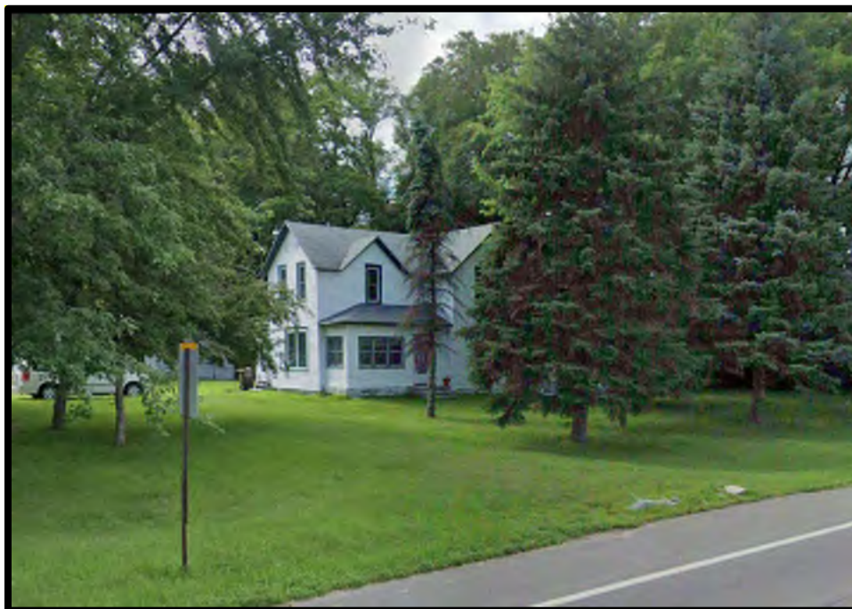
View of HE-COC-006 showing the façade of the building.
