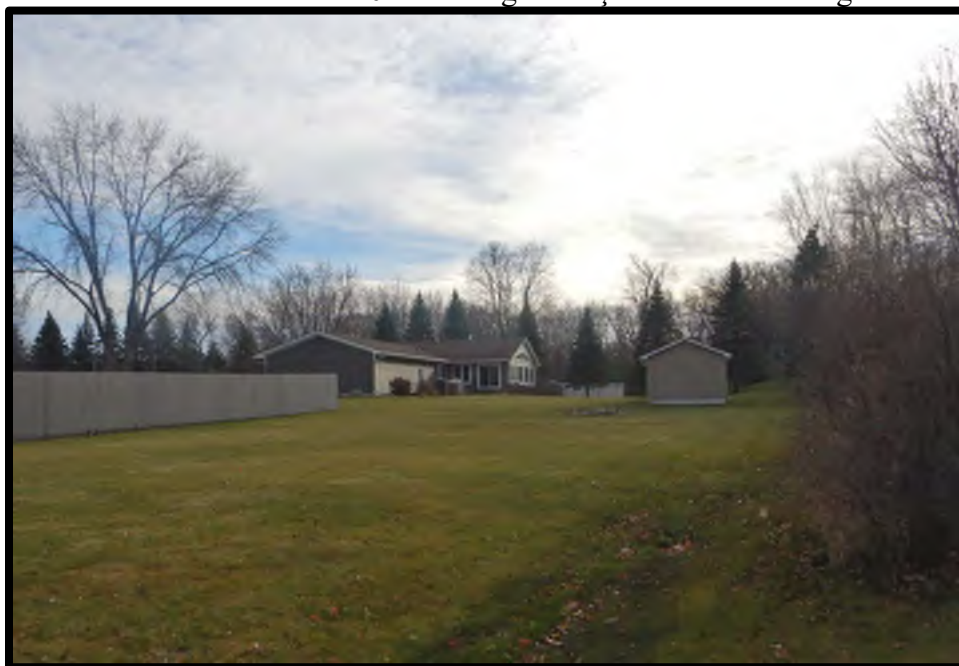
View of FLDNUM 02 showing the rear of the building.
