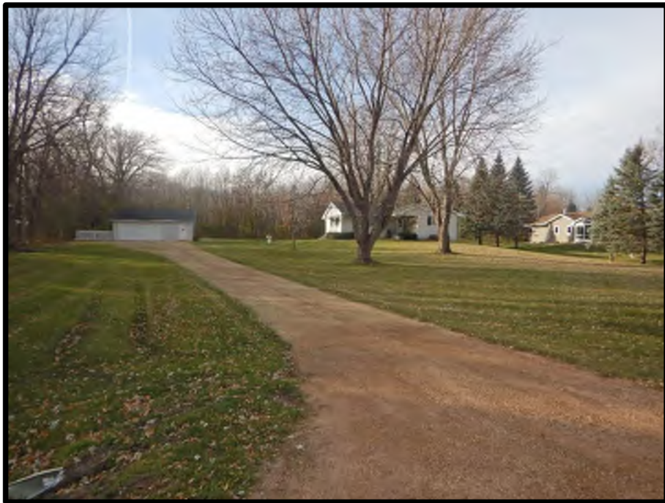
Figure 12. View of FLDNUM 01 showing the façade of the building and the garage.
