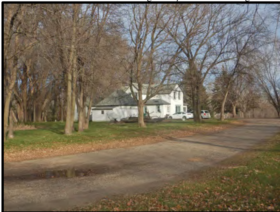
View of HE-COC-006 showing the rear of the building and remaining outbuildings.
